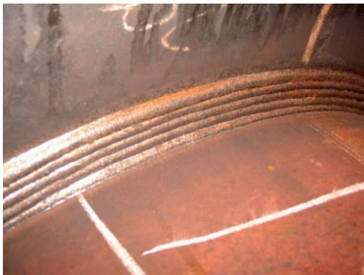
写真-10 溶接外観
